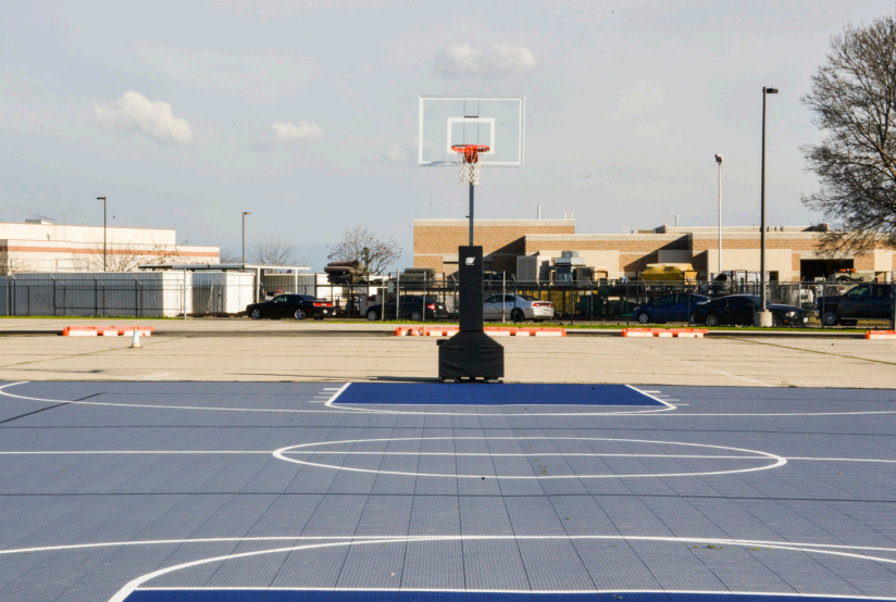
The 144th Civil Engineering Squadron assisted the Force Support Squadron with their recent purchase of an outdoor basketball court by laying a level foundation for the court. (Air National Guard photo by Capt. Jason Sanchez)
